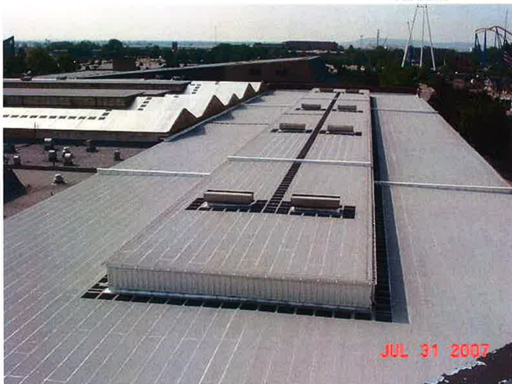
KENTUCKY EXPOSITION CENTER WEST WING PAVILION Louisville, KY
