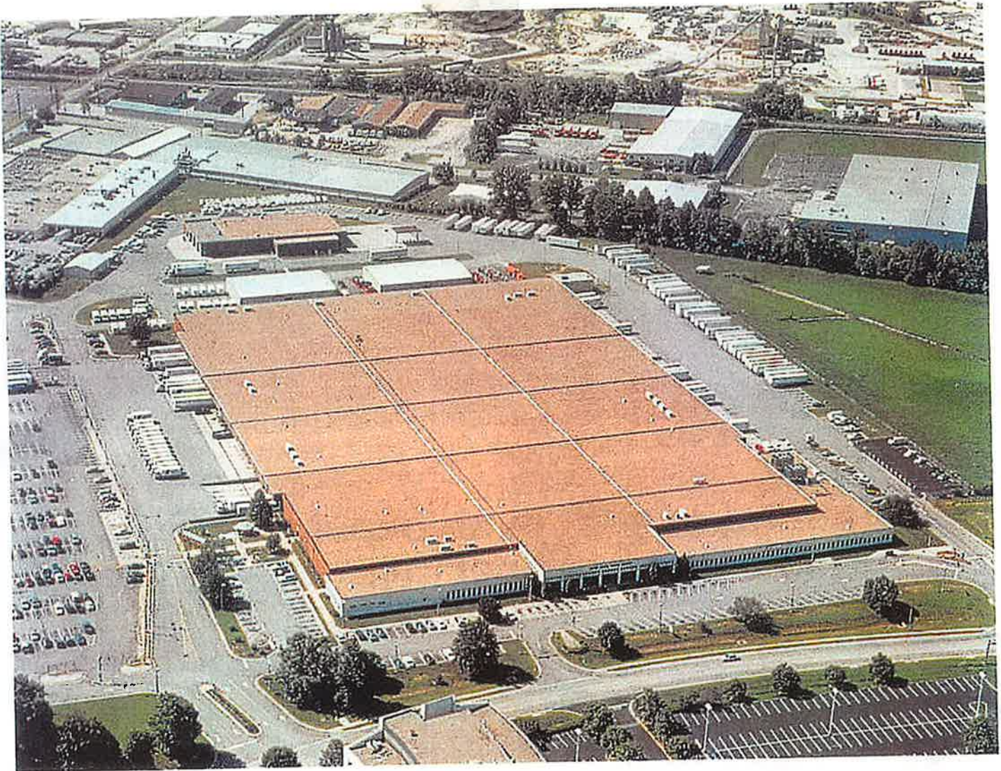
This postal facility in Kentucky is surfaced with almost 43,000 m 2 of Paradiene cold-adhesive applied membranes.
